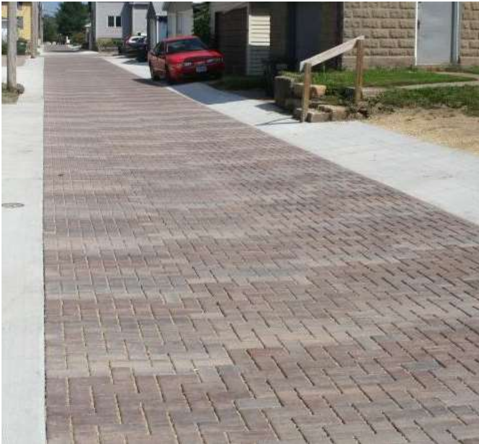
Motor vehicle space is clearly defined through use of materials and pattern.
